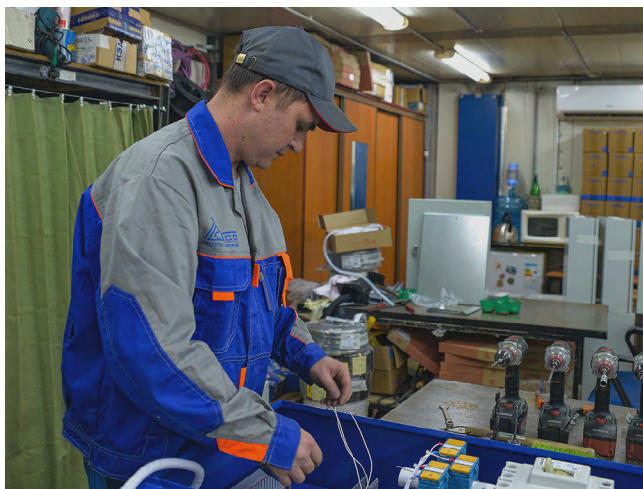
ASSEMBLY OF CONTROL BOARDS
